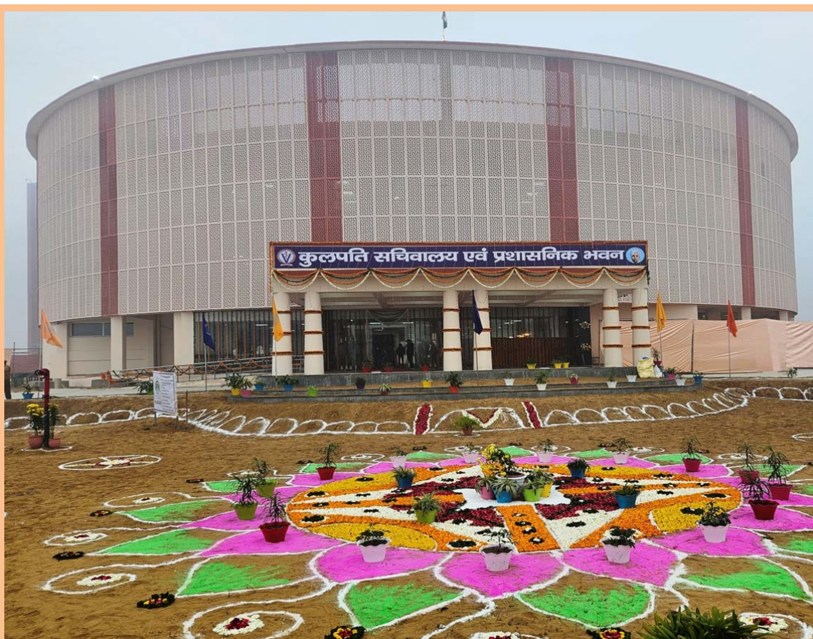
Administrative Block, New Campus, LUVAS
